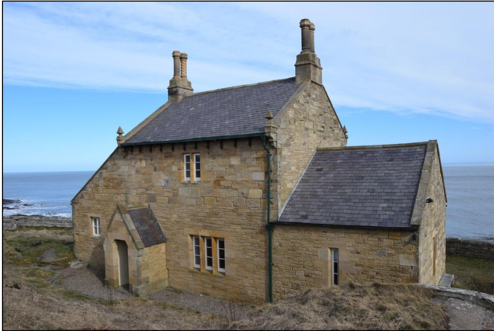
Fig 3: The Bathing House, view to the Northeast
