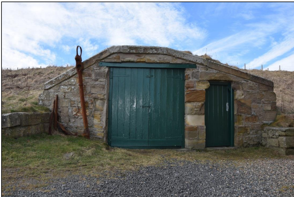
Fig 4: The Listed outbuilding, possibly a 'coach house', view to the west
