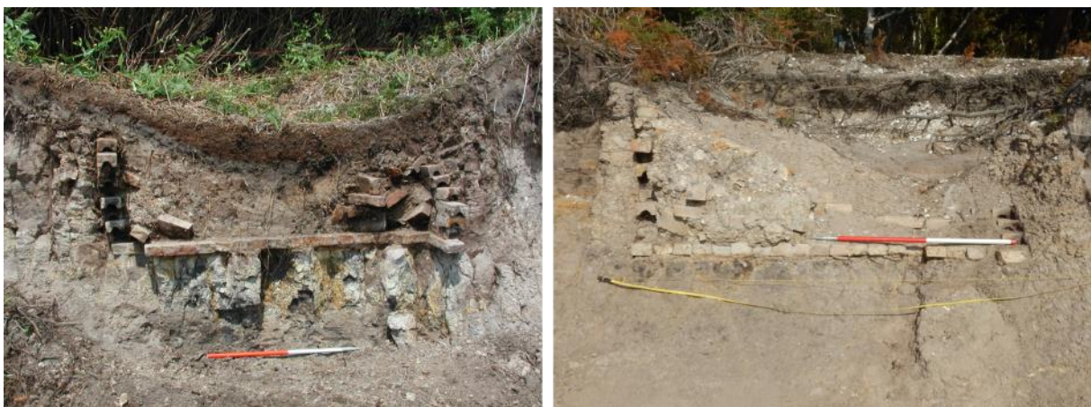
Figure 26 Left: Photograph of the Brick Lined Tank in 2005 (National Trust). Right: Photograph of the Brick Lined Tank 2016.
