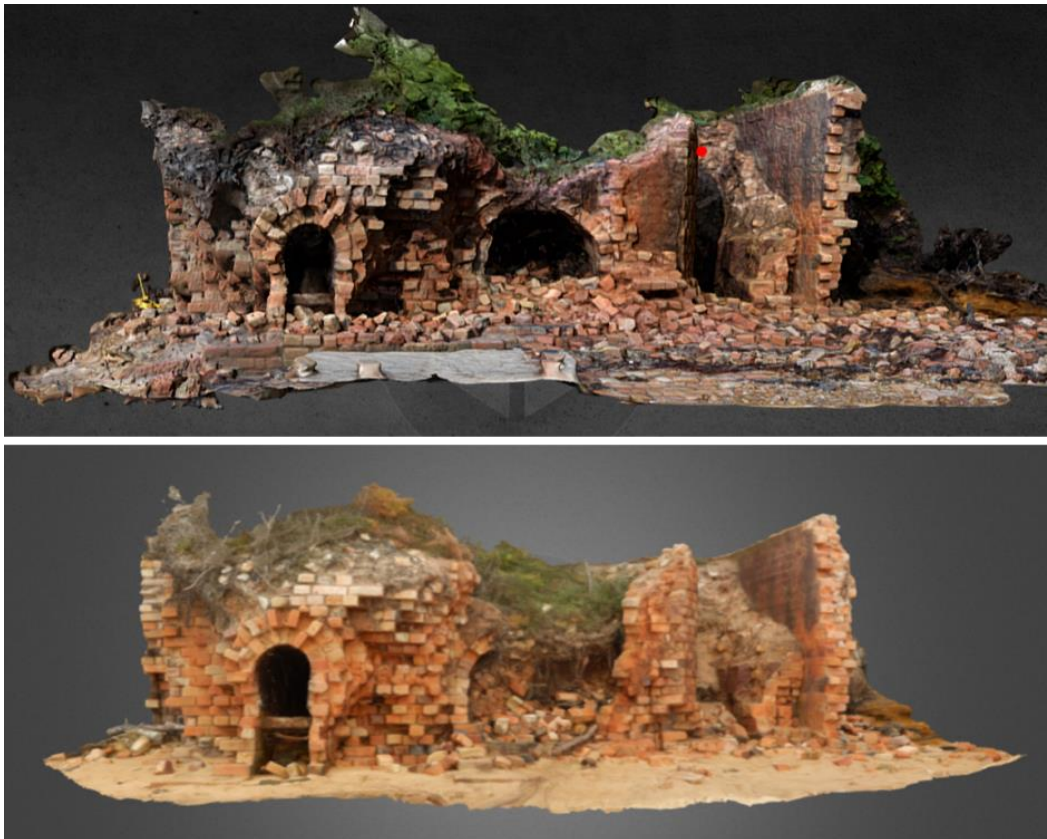
Figure 23: Comparison of the 2015 3D model of Barnes Brick Kiln (top) with the 2016 model (bottom). The main brick lined kiln has collapsed in the time between the models being created.
