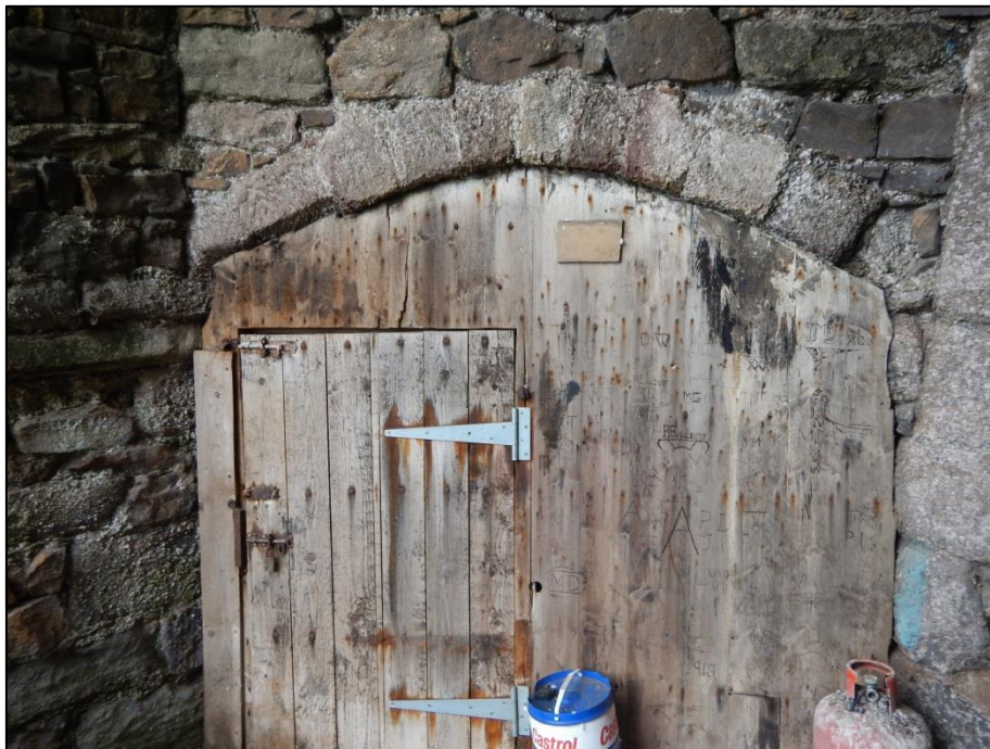
Fig 17: Door to converted storeroom inside Beadnell Harbour limekiln
