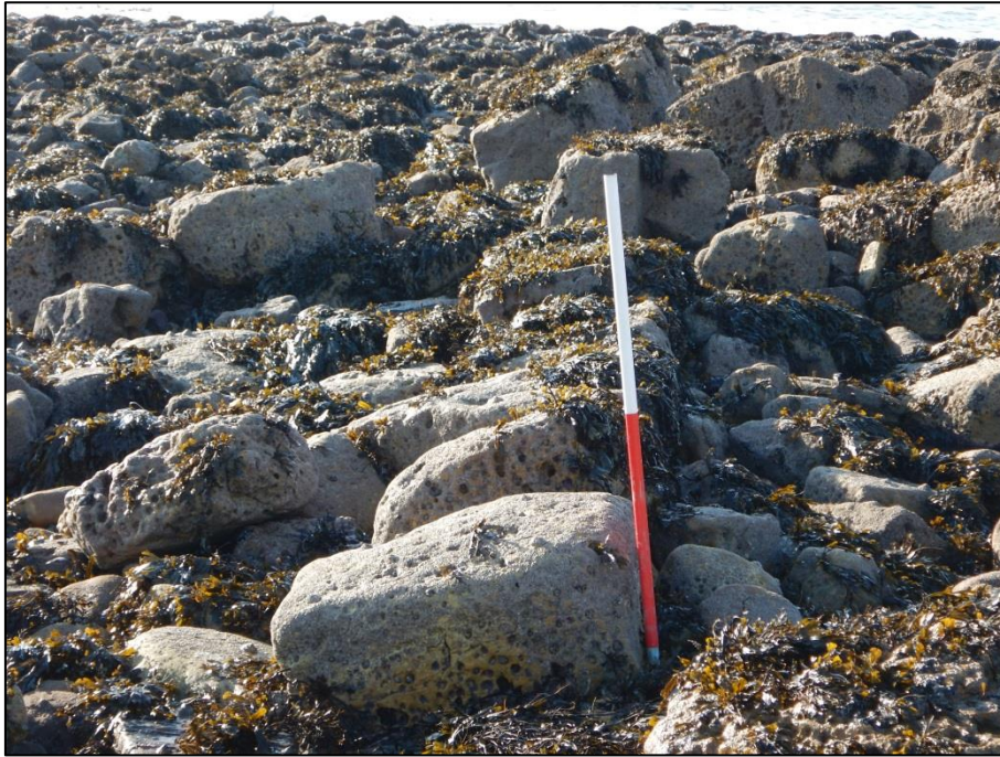
Fig 14: Detail of lowest course of the possible pier
