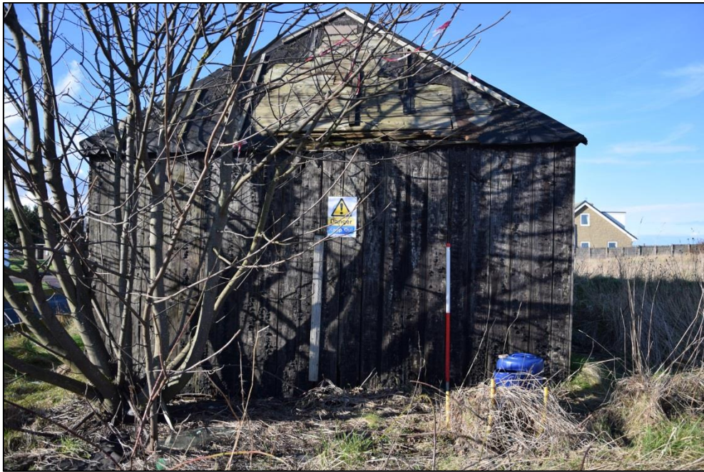
Fig 9: South facing in elevation of fisherman's hut
