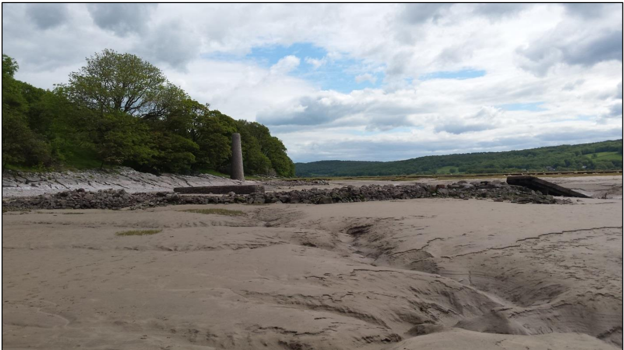
Figure 8: The foreshore at Jenny Brown's Point, showing the collapsed bridge (foreground), the small stone quay (PRN 520; middle ground) and chimney (UID 181949/PRN 4821; background). View to the northeast.
