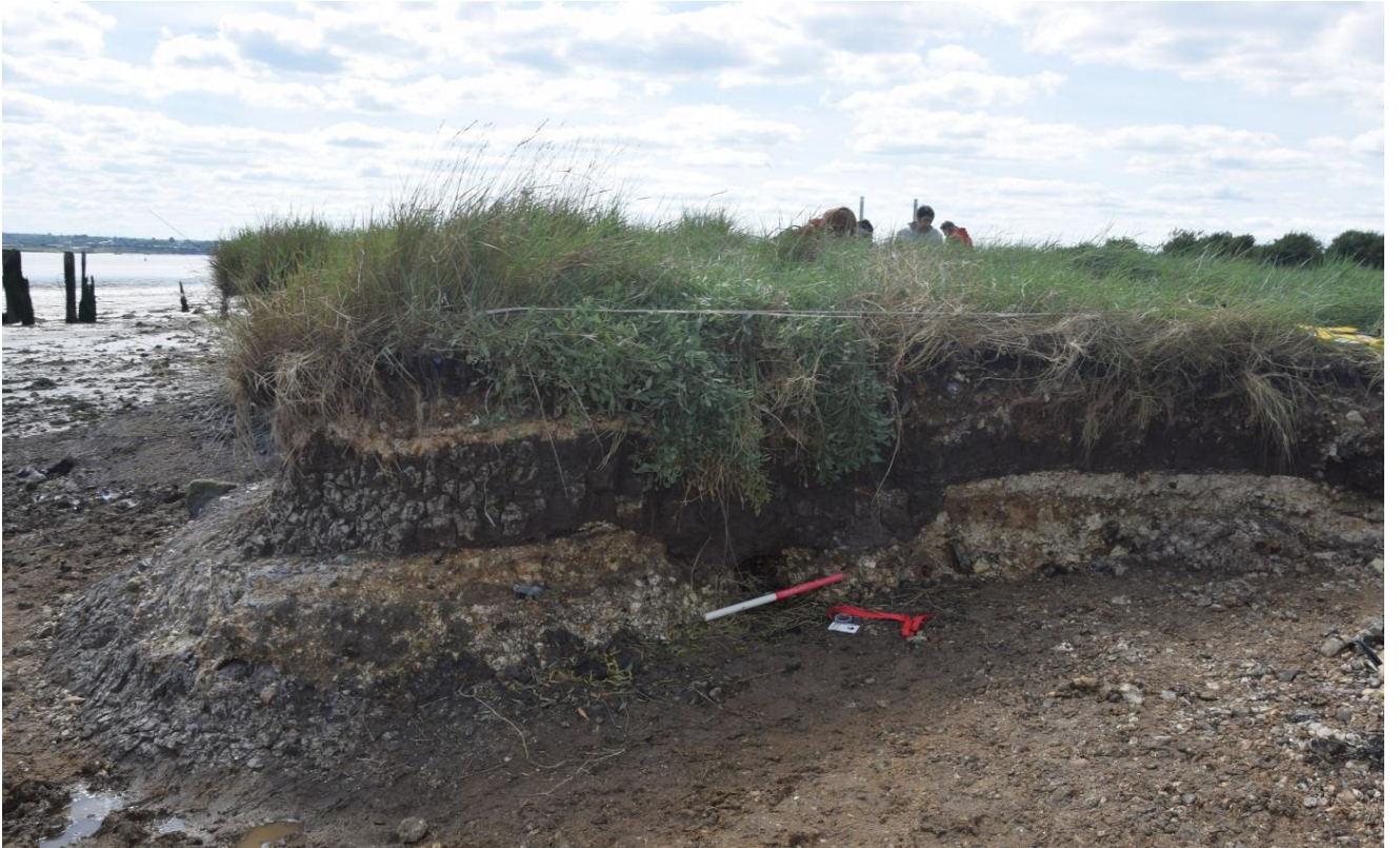
Figure 14 Area 3: made ground
