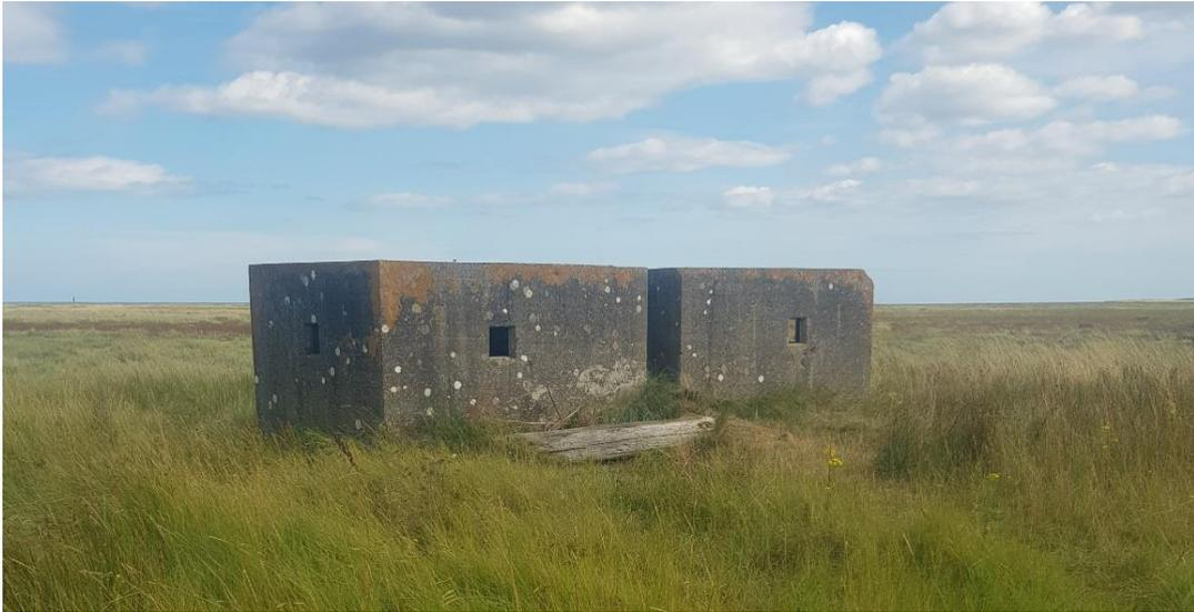
The pillbox, often incorrectly referred to as a 'bunker', is the archetypal structure of First and Second World War defences in the UK. These often small structures are constructed from reinforced concrete, and feature embrasures within their walls to allow the occupants to fire a variety of weapons from the relatively safe confines of the pillbox.
