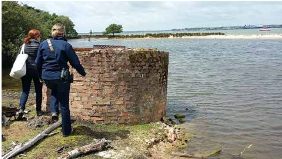
Figure 35 One of several shafts associated with the clay industry on Brownsea Island.
