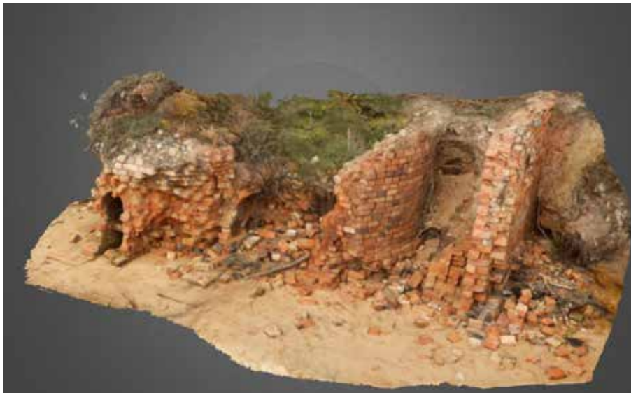
Figure 22 3D model of the Brownsea Brick Kiln, in 2016 showing erosion. Note the collapsed arch, centre.
